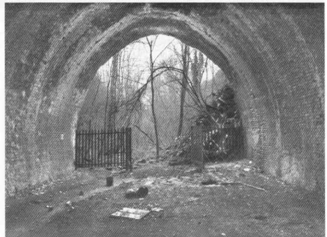
The north portal of Etchinghill Tunnel in March 2012
